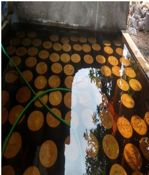
Perawatan Beton (Curing)
