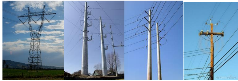
Gambar 2.3 Jenis Tower: (a) Lattice Tower , (b) Tubular Steel Pole , (c) Concrete Pole , dan (d) Wooden Pole
