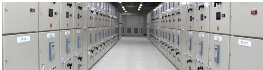
Gambar 2.6 Switchgear
