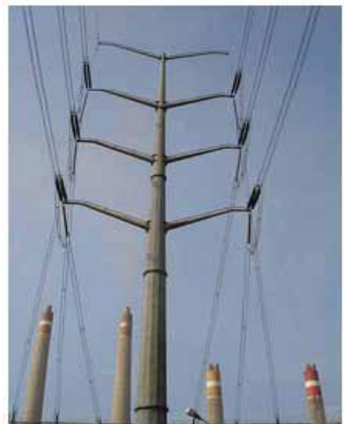
Gambar 2.10. Tiang Saluran Tubular Steel Pole
