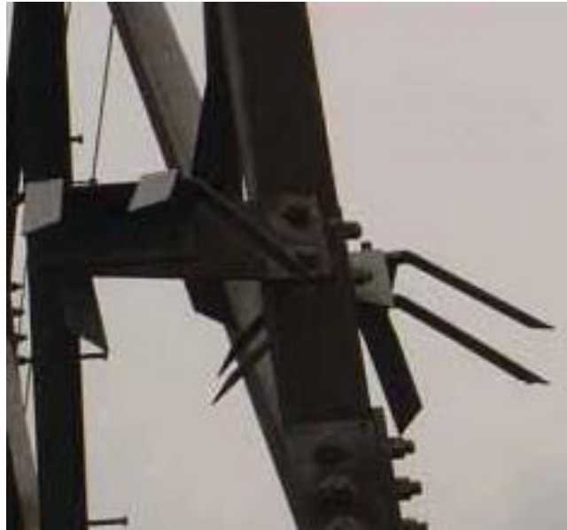
Gambar 2.17. Anti Climbing Device (ACD)
