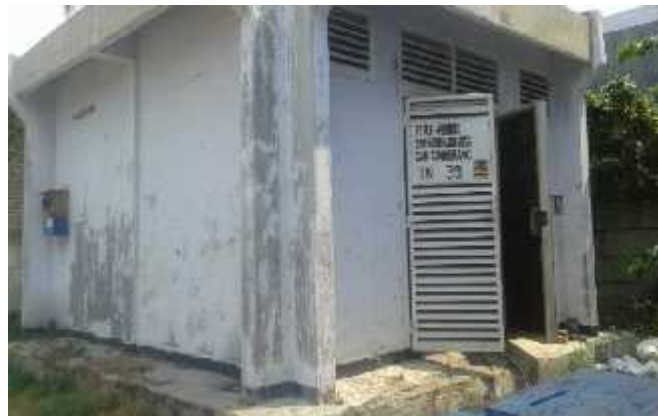
Gambar 2.8 Gardu Distribusi Tipe Beton
