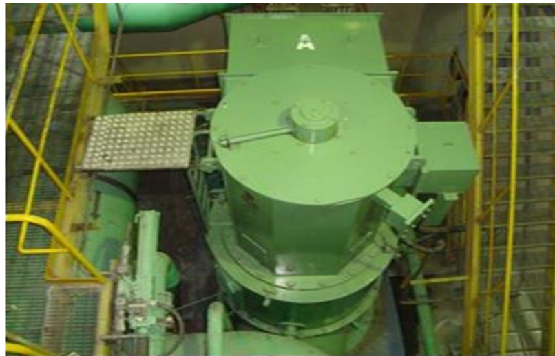
Gambar 2.10 Main Cooling Water Pump
