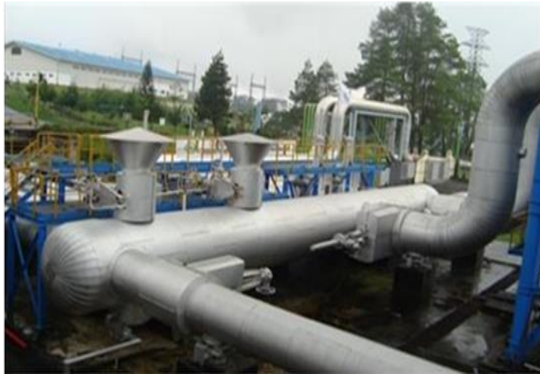
Gambar 2.2 Steam Receiving Header
