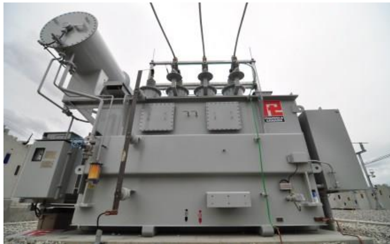
Gambar 2.18 Generator Transformer/Transformator
