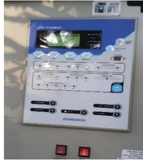
Gambar 2. 7 Remote Terminal Unit (RTU)
