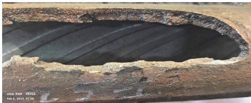
Gambar 2. 13 Kegagalan Hydrogen Damage
