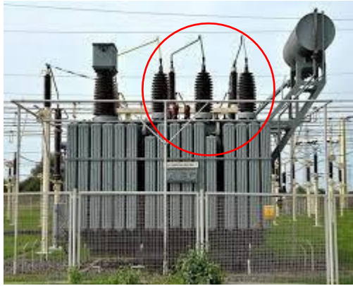
Gambar 2.5 Bushing trafo
