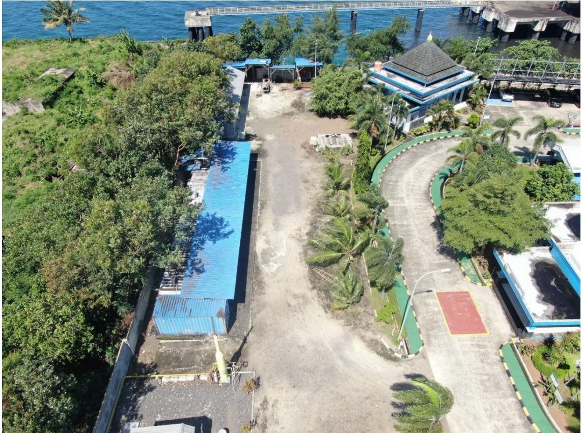
Gambar 4 24 Kondisi Aerial View- Area Pergudangan
