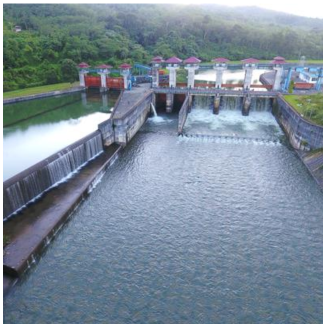
Gambar 3. 2 Intake Dam PLTA Musi
