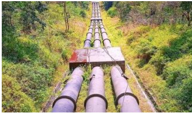
Gambar 2 6 Pipa Pesat (Penstock) ( https://www.shutterstock.com/id/search/penstock-pipe )
