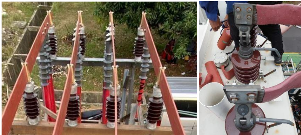
Gambar 2. 4 Design Busbar 20kV Terbuka
