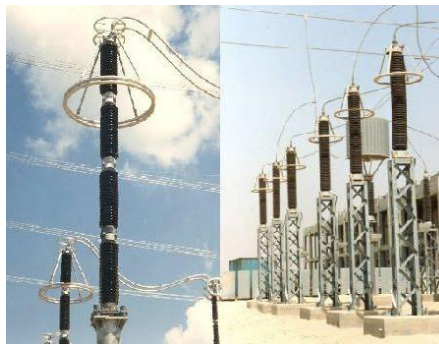
Gambar 2. 4 Lightning Arrester
