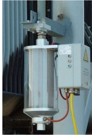
Gambar 13 Dehydrating Breather
