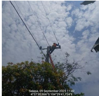
Gambar 3.4 Proses Pemasangan Protective Sleeve
