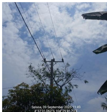
Gambar 3.5 Sesudah Pemasangan Protective Sleeve
