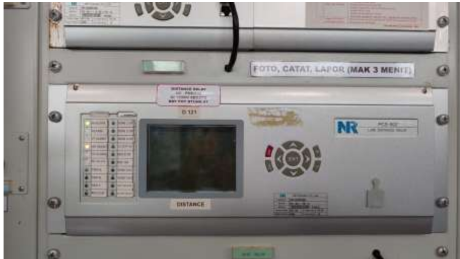
Gambar 2. 2 Rele Jarak (Distance Relay)
