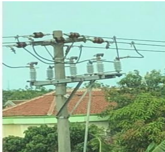
Gambar 17 LBS (Loaad Break Switch) Manual
