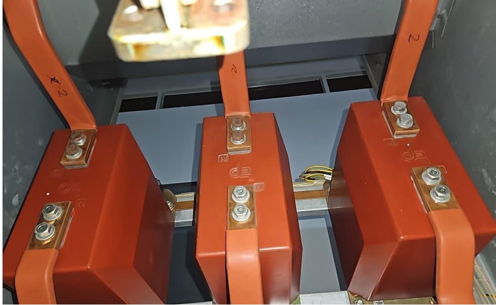
Gambar 2. 4 Current Transformer (Trafo Arus)
