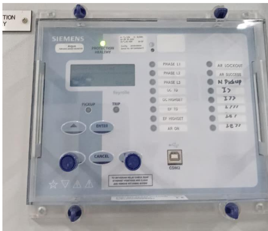
Gambar 2. 1 Over Current Relay
