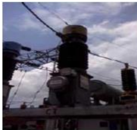
Gambar 2. 6 Transformator Arus
