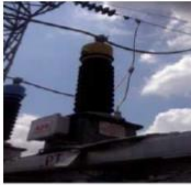
Gambar 2. 7 Transformator Tegangan
