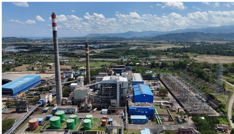
Gambar 2. 1 PLTU IP UBP Barru 1x100 MW
