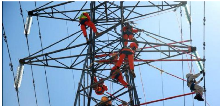
Gambar 2. 4 PDKB TM Methode potensial
