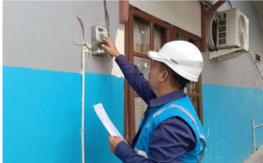
Gambar 2.3 Pergantian kWh meter
