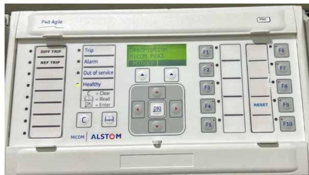
Gambar 2.4 Relay Differential MICOM P643 Numerik
