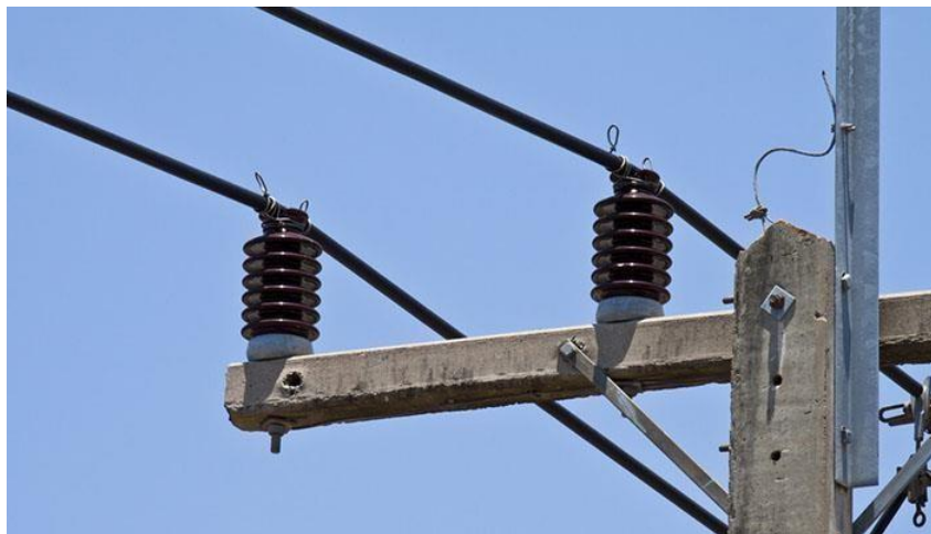
Gambar 2.2 Isolator Post (sumber : www.hbjinyong.com/id/insulator/post-insulator/ )
