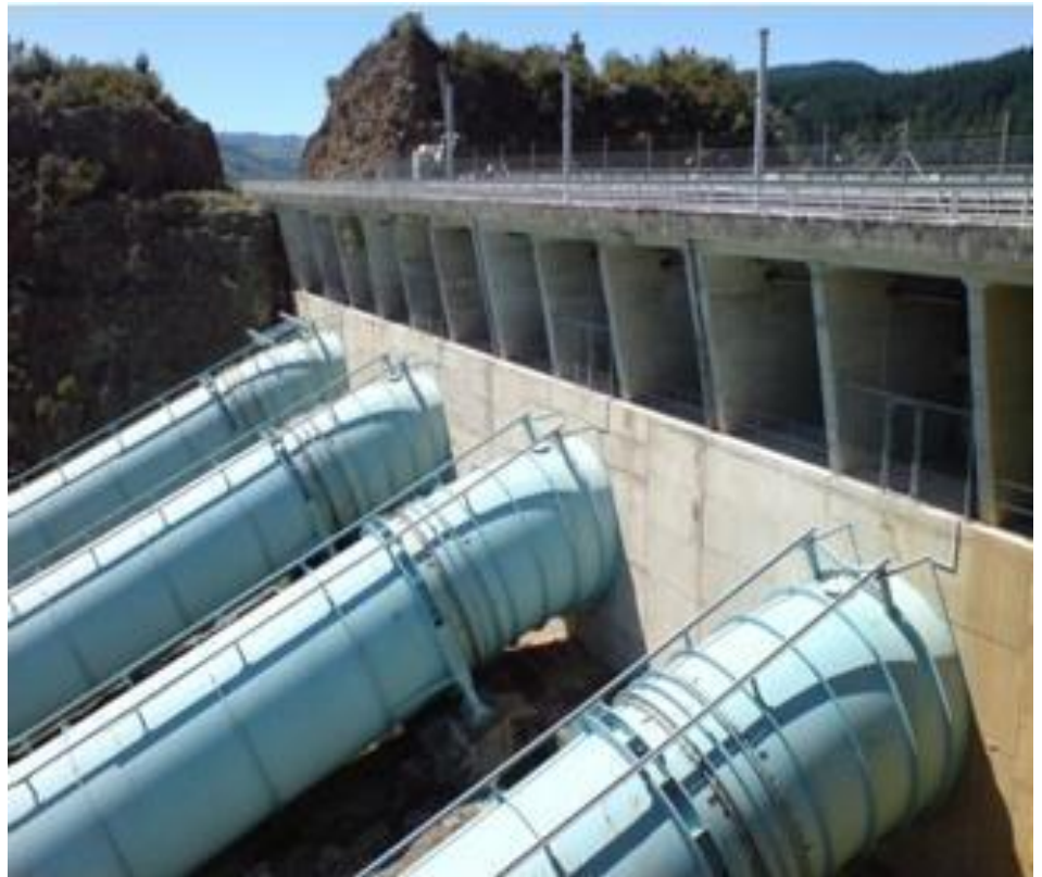
Gambar 2.4 Pipa Pesat ( Penstock )
