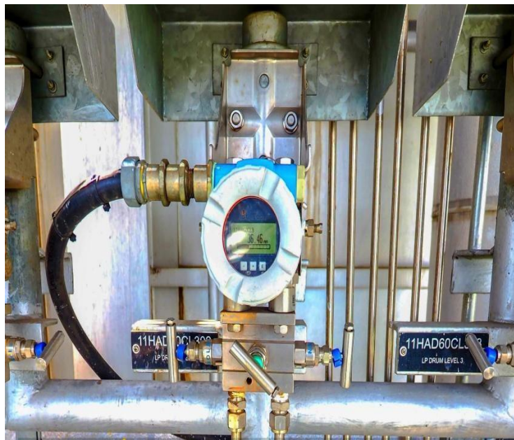
Gambar 2.13 Differential Pressure Method
