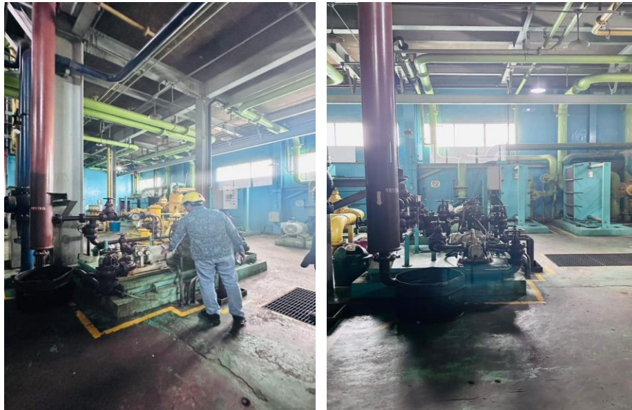
Gambar 2.3.4 Sistem Pelumasan ( Lubricating System )
