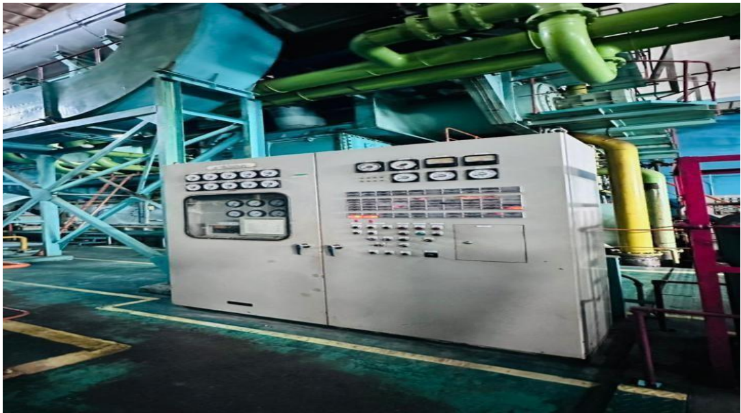
Gambar 2.3.7 Sistem Pengendalian & Pengaman ( Governor System )
