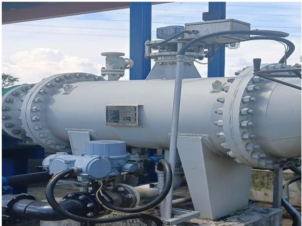
Gambar 2. 22 Screen Debris Filter
