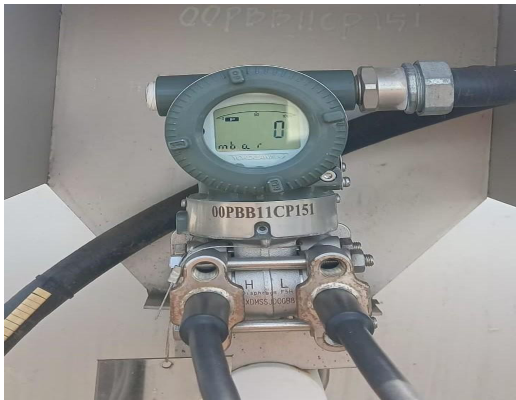
Gambar 2. 25 Differential pressure transmitter
