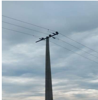
Gambar 2. 7 Tiang Beton JTM
