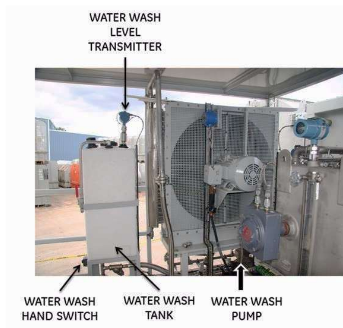
Gambar 2.17 Perlengkapan Water Wash Compressor
