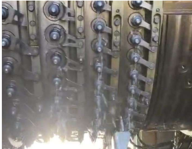
Gambar 2.18 Witness dan Pengambilan Sampel Water Wash Compressor
