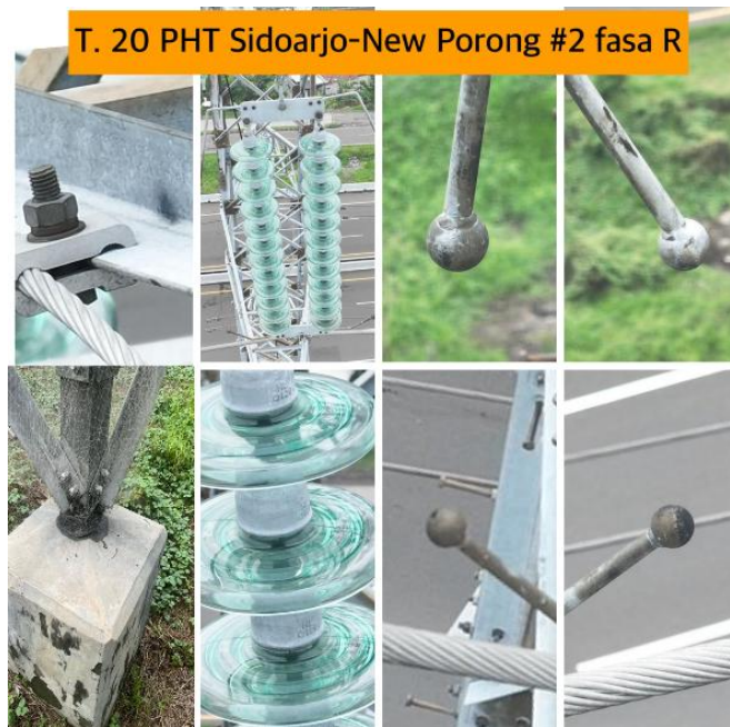
Gambar 4.9.6 Hasil CUI Isolator dan Fitting
