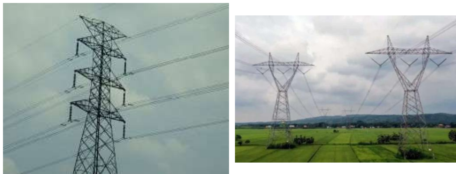
Gambar 2.10 a. Zig-zag Tower & b. Tiang Delta (Delta Tower)
