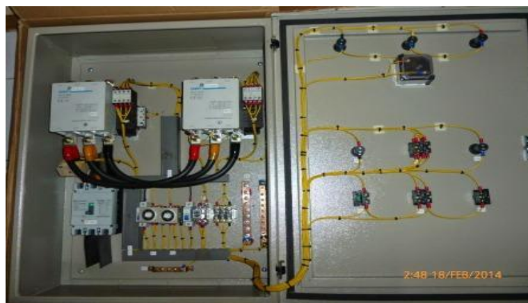
Gambar 2.3 Contoh Panel ACOS (Automatic Change Over Switch)
