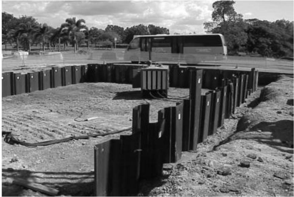
Gambar 2.5 *Sheet Pile Wall*
