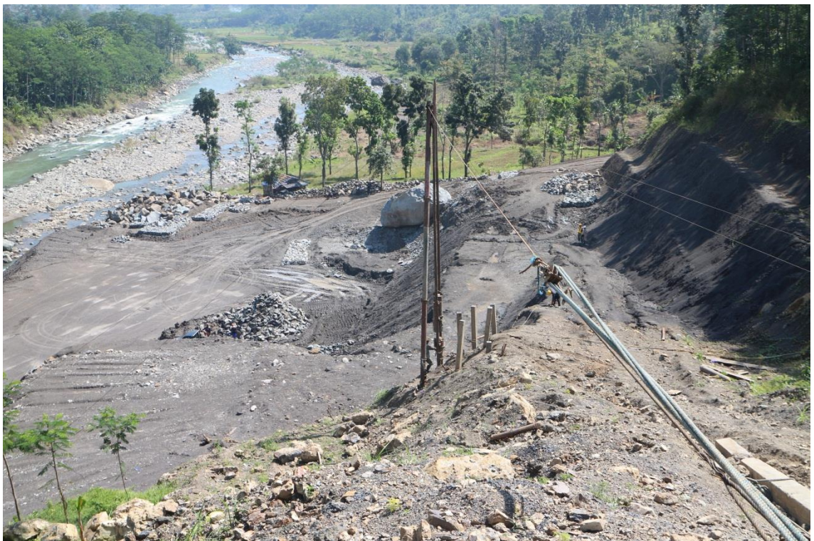
Gambar 6.3 Lokasi Power House
