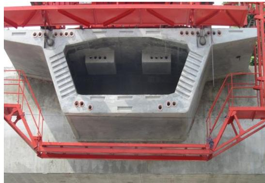
**Gambar 2.13** Setelah cor kemudian Buka bekisting, *Curing, Stressing+ Grouting*
