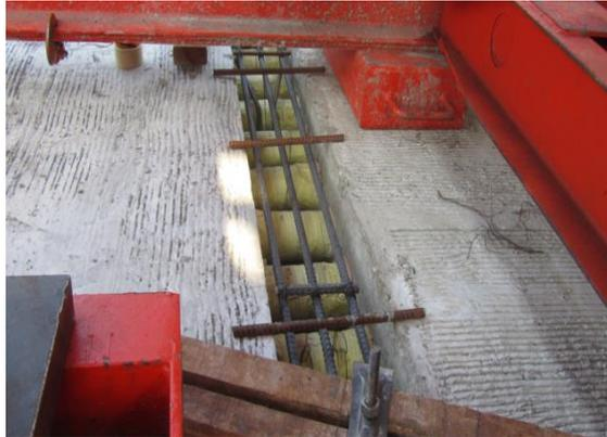
**Gambar 2.12** Sambungan *ducting tendon*
