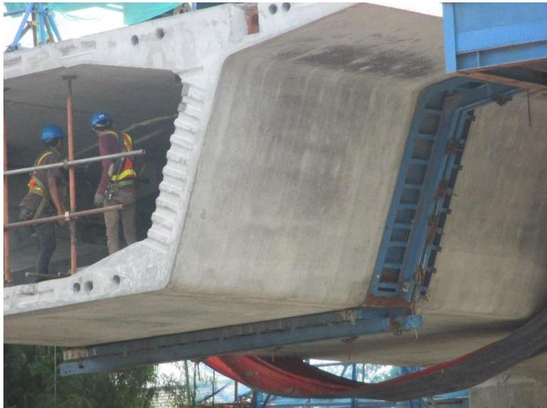
**Gambar 2.51** *Wetjoint* Yang Sudah Terpasang *Formwork*
