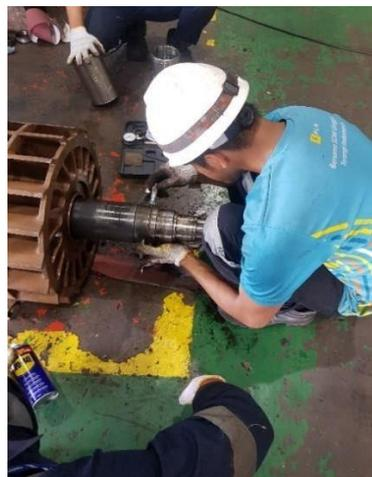
Gambar 4.10 Diameter Inspection
