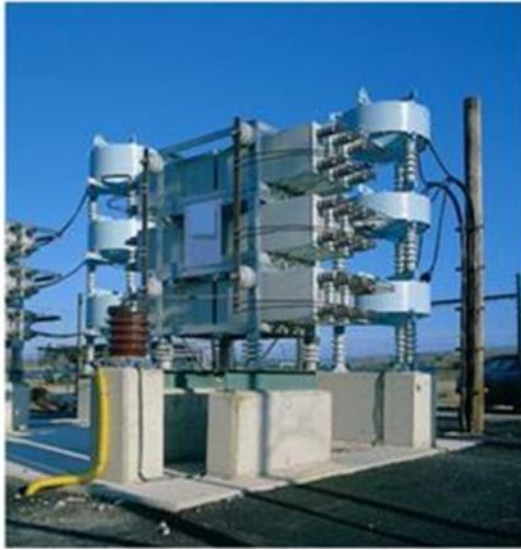
Gambar 2.3. Kapasitor Filter
