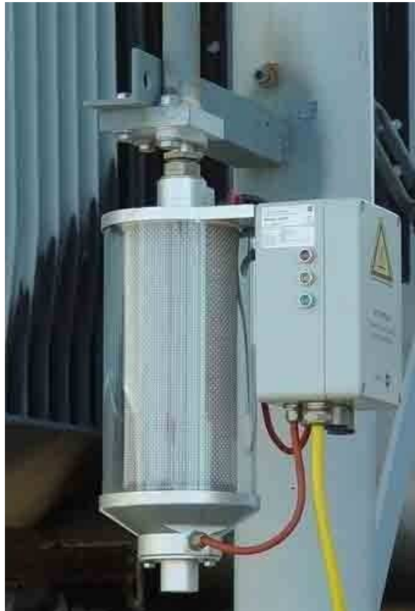
Garmbar 2.15 Alat Bantu Pernapasan ( Dehydrating Breather )
