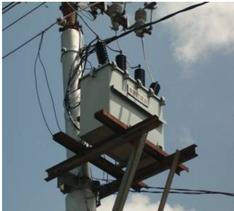
Gambar 2.19 Transformator Instalasi Gardu Cantol
