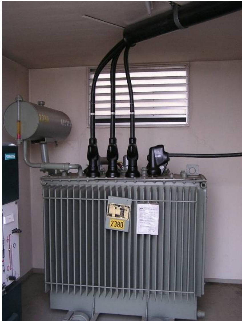
Gambar 2.17 Transformator Instalasi Gardu Beton
