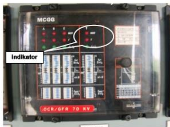
Gambar 2.15 Relay Arus Lebih (Over Current Relay)
