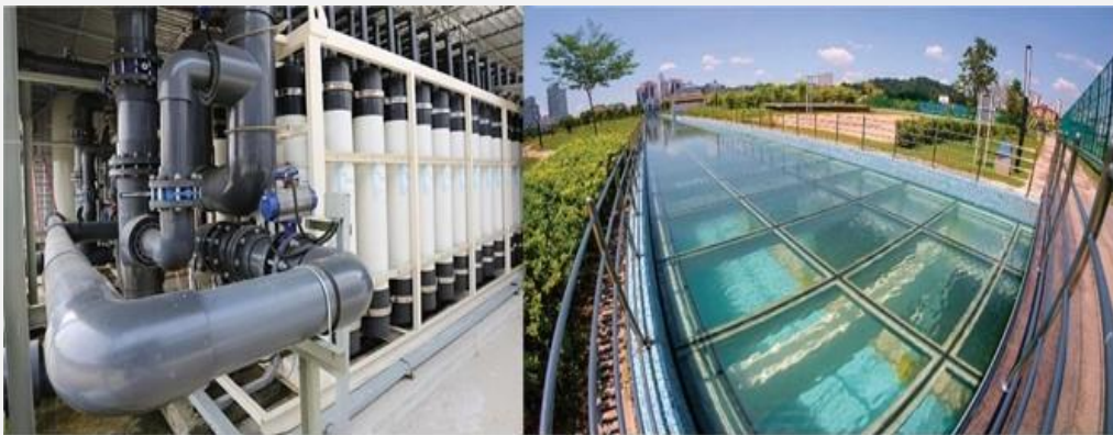
The Pantai Dua WWTP features ultrafiltration units and an aquatic skylight.
