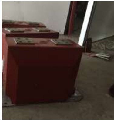
Gambar 2.14. Transformator Arus (CT)
