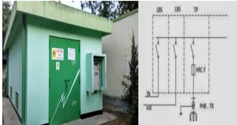
Gambar 2.1 Gardu tembok dan single line diagram
