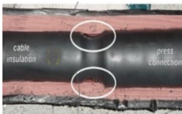
Gambar 2.2 Cavities in the shrink type cable joints
