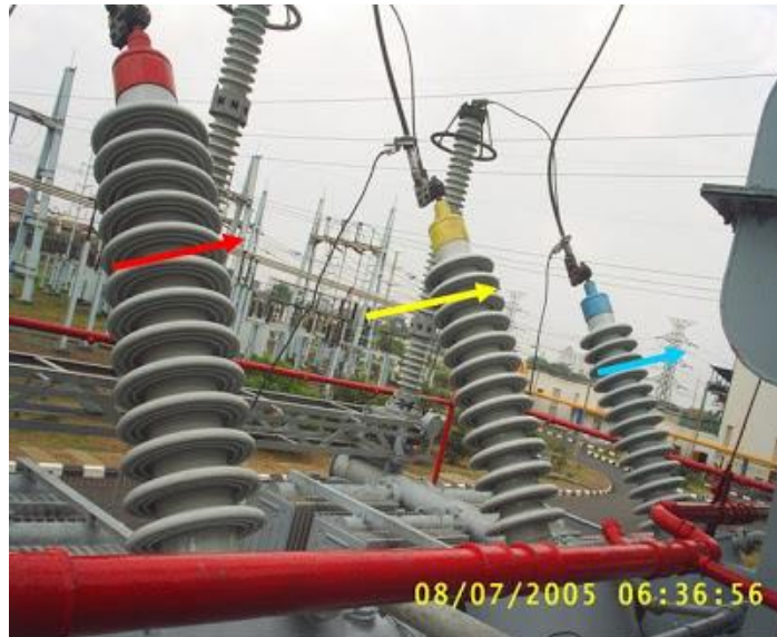
Gambar 2.5 Bushing Tranformator
