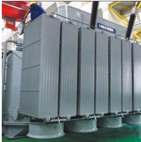
Gambar 2.6 Radiator Transformator
