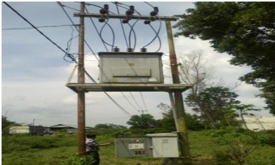
Gambar 2.7 Pole Mounted Circuit Breaker
