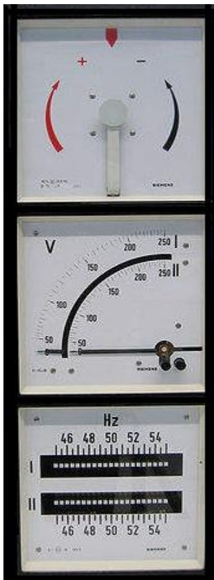
Gambar 5. 41 Peralatan Sinchron
