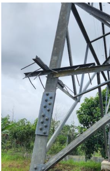
Gambar 2.10 Anti Climbing Device (ACD)
