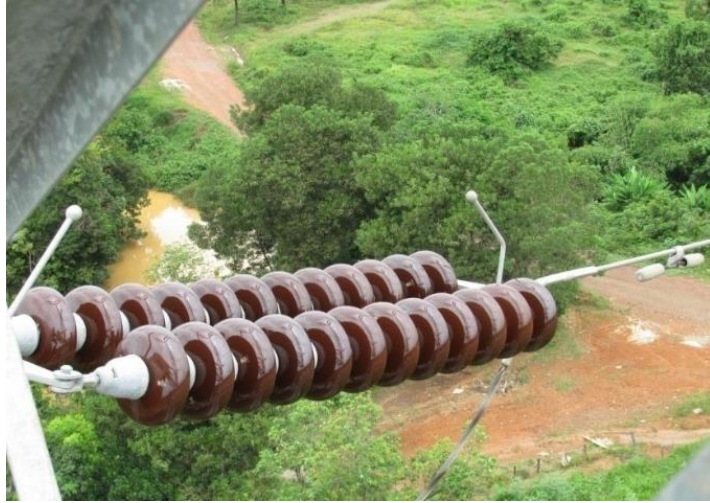
Gambar 2.2 Ceramic Insulator
