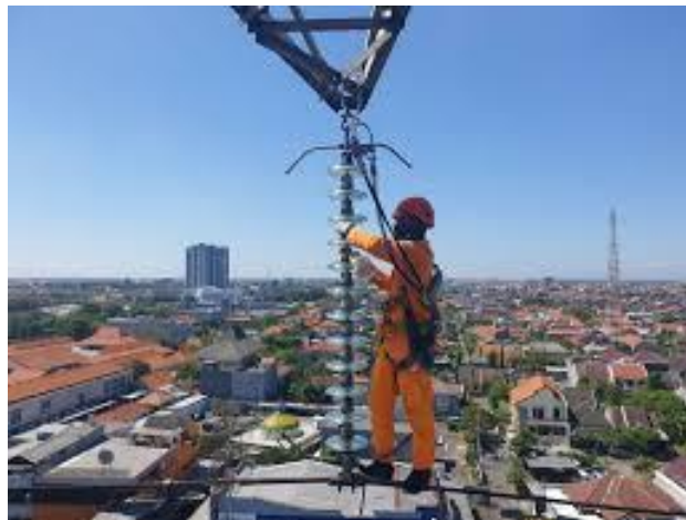
Gambar 2.16 Penambahan Keping Isolator
