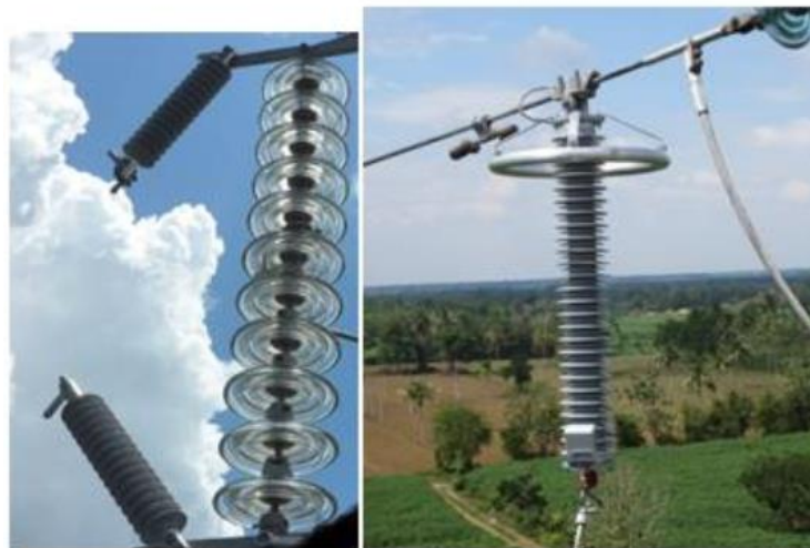
Gambar 2.20 Transmission Line Arrester
