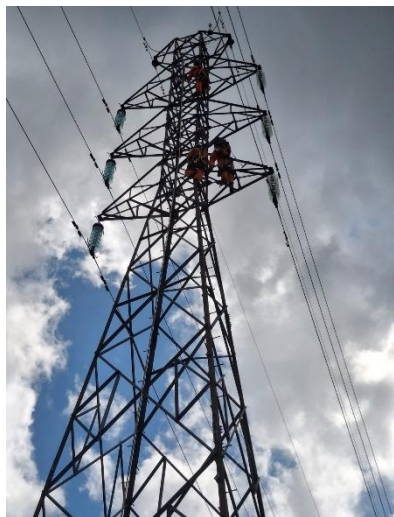
Gambar 2. 4 Tower suspension (dokumentasi pribadi)
