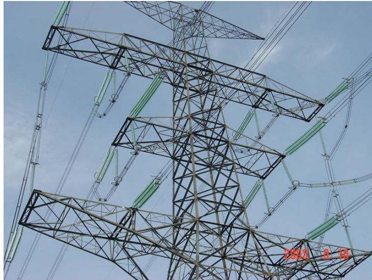
Gambar 2. 5 Tower transposisi [20]
