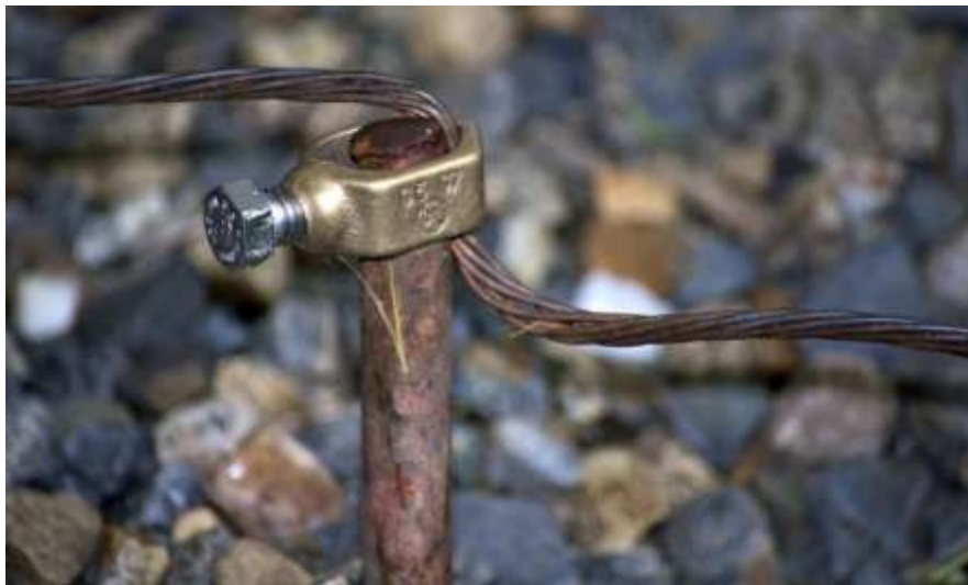
Gambar 2.2 Rod pentanahan ( Grounding )
