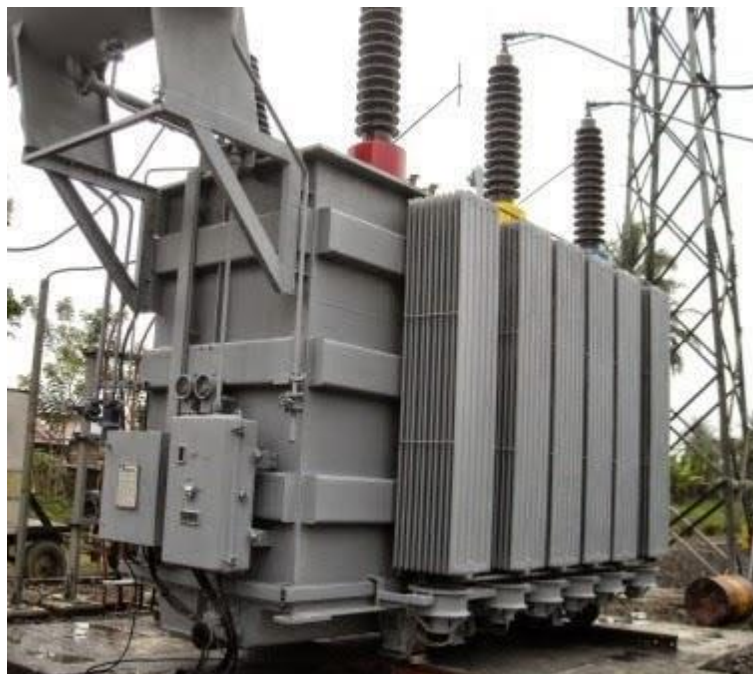
Gambar 2. 4 Transformator Daya
