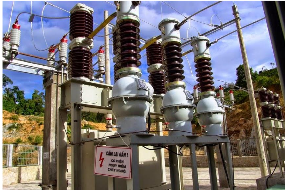
Gambar 2. 6 Current Transformer
